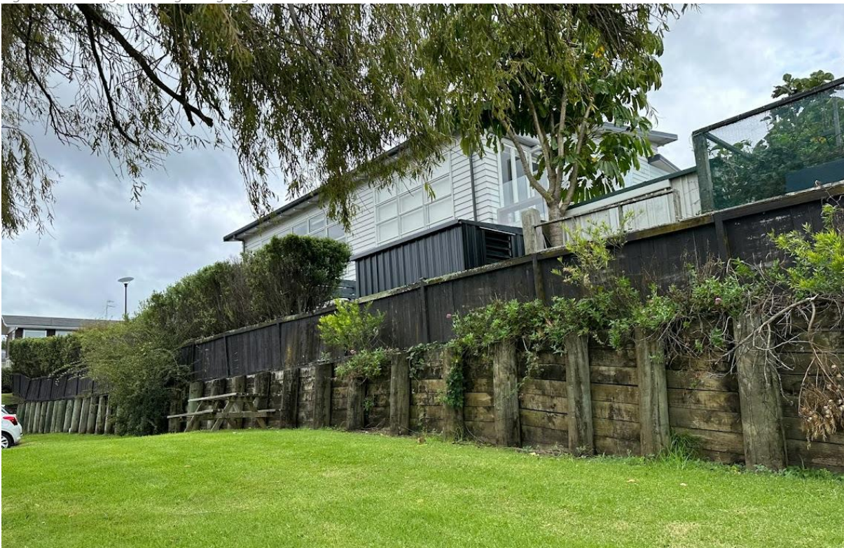
Figure 4: Existing retaining along Pigeon Mountain Road.
