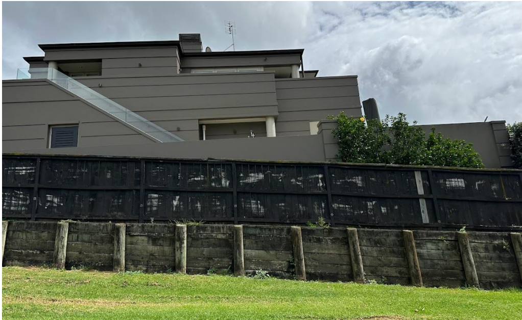
Figure 10: Adjoining property to the west.
